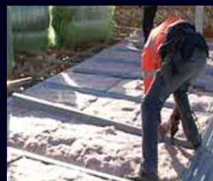
Many spacer battens secured
