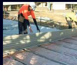
Roof sheet is then tacked in place
