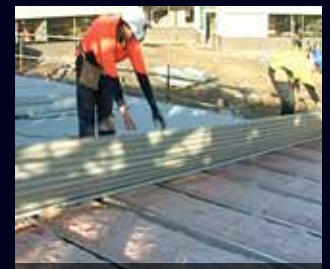
Roof sheet is then tacked in place
