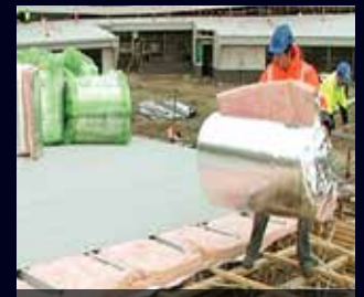
Insulation rolls are "man-handled"
