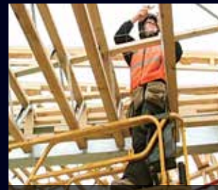
Painstakingly labour intensive wire
