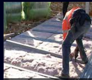
Many spacer battens secured
