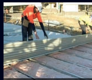
Roof sheet is then tacked in place
