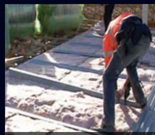
Many spacer battens secured
