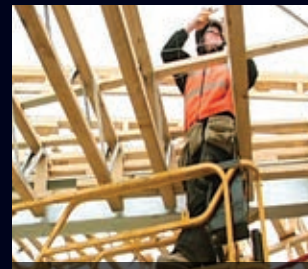
Painstakingly labour intensive wire
