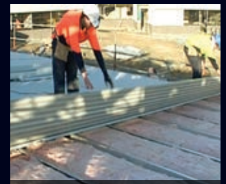
Roof sheet is then tacked in place
