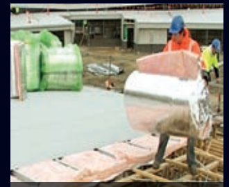
Insulation rolls are "man-handled"
