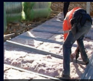
Many spacer battens secured
