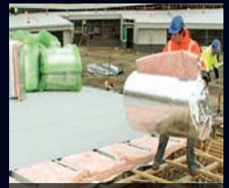
Insulation rolls are "man-handled"
