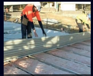
Roof sheet is then tacked in place
